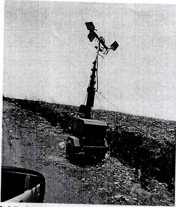
Mobile Lighting System at Deonar Dumpsite
